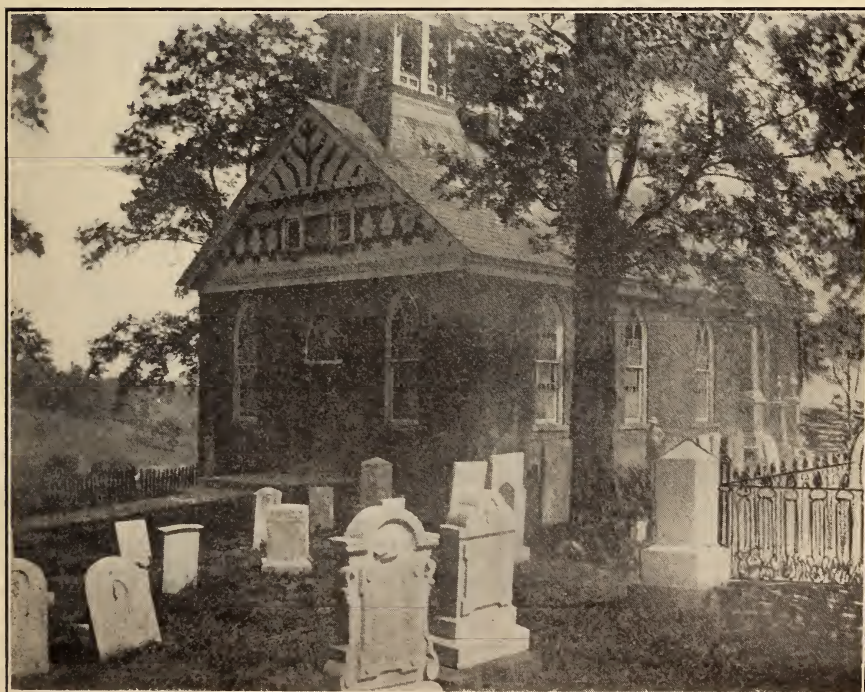
ST. JOHN'S CHURCH, EAST SPRINGFIELD, BUILT 1833.
